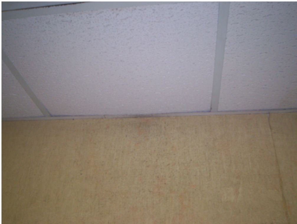
Photograph 2 —GRU Operation Center office space. Staining was noted on the wallpaper in the break room.
