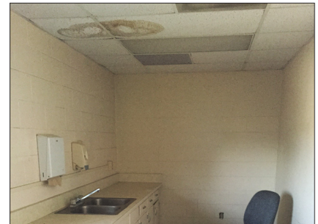
Water Damaged Ceiling Tiles
