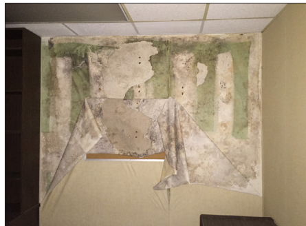
Mold Growth On Interior Wall
