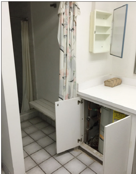
Toilet Room With Under-Counter Water Heater
