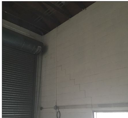
Wall Cracking
